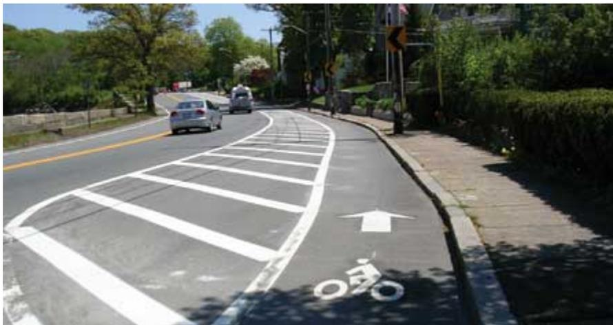
**Figure 1:** A Complete Street approach provides provisions for bicycles (a bike lane in this case), pedestrians, and vehicles – all within the same right-of-way.
